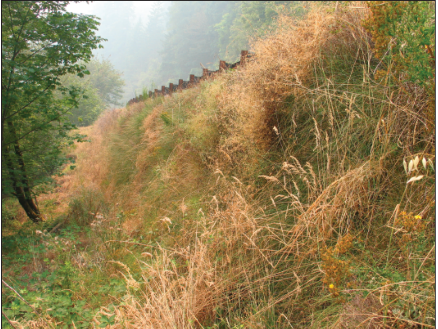
Three years after installation, native grasses are well established on 20 feet high soil faced retaining walls.
