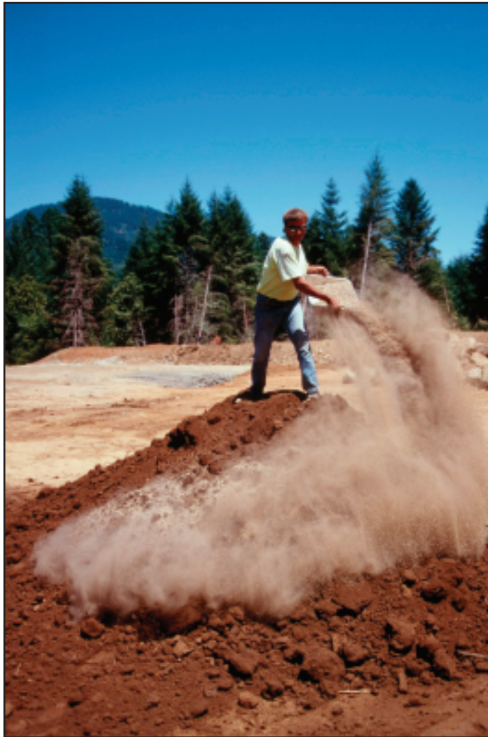
Topsoil was manufactured on site using loam from an alluvial deposit and mixing it three bucket loads of loam to one bucket of compost. Lime, slow release fertilizer, and mycorrhizae were added and then thoroughly mixed in.
