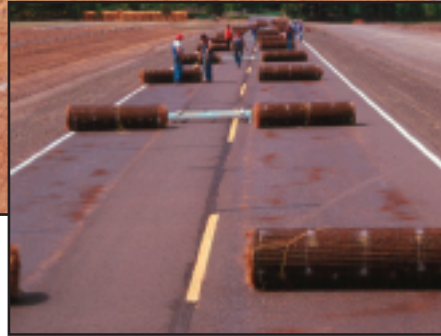
Seeds were sown on erosion mats and glued to the surface. After the glue dried, the mats were rolled up and stored until construction of the walls.
