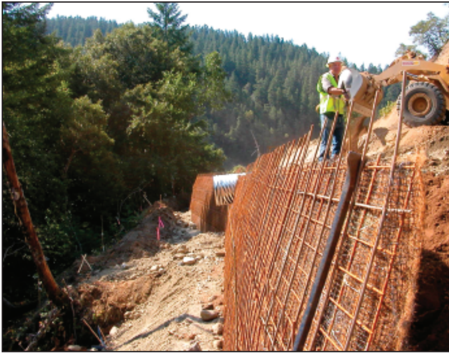
As retaining walls were built, seeded mats were attached to the frames and filled behind with a foot of topsoil.
