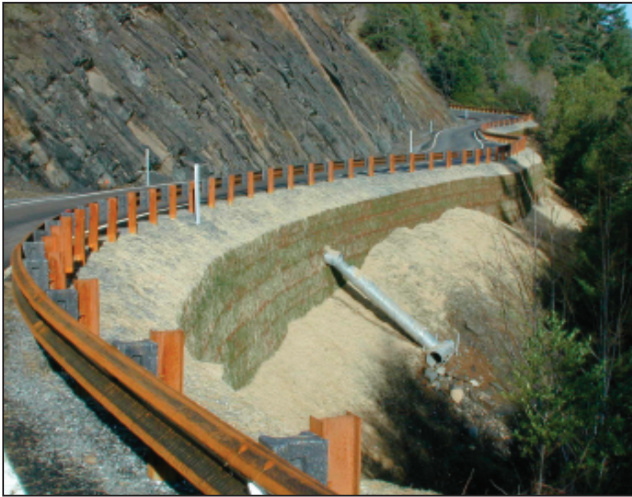
Above: 2003. Grass seeds began to germinate in late fall, three months after wall installation. Below: 2006. Three years later, retaining walls are screened by strands of native grasses.
