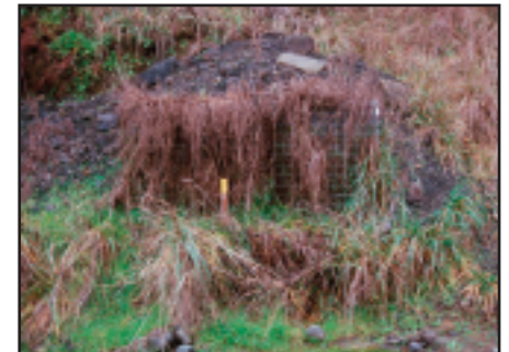
The first year experiment to establish grasses on soil-faced walls failed as a result of poor topsoil and annual weeds. The findings from our test plots proved invaluable for the final project.
