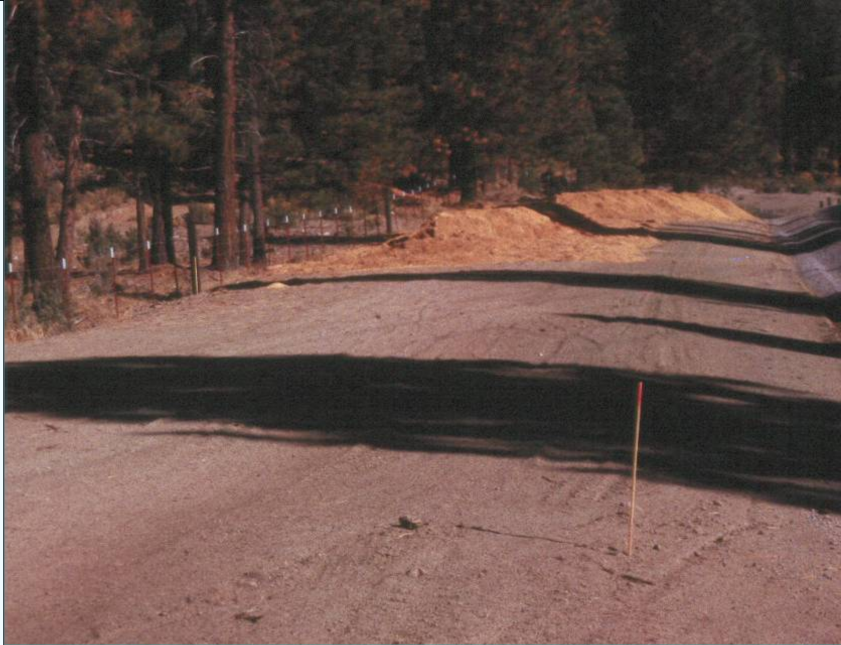
Truckloads of Medite were placed on the abandoned road surfaces, then spread with a tractor to achieve an approximate 4" mulch depth.
