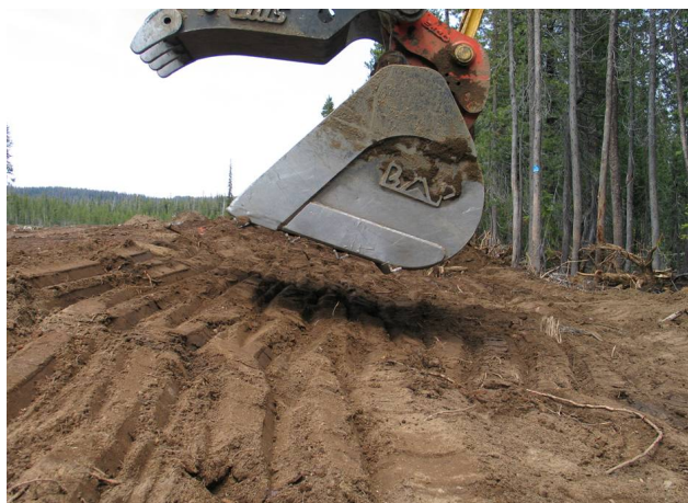
Figure 3. Bucket imprinting uses the face of an excavator bucket to create a roughened soil surface similar to trackwalking but with significantly less soil compaction.
