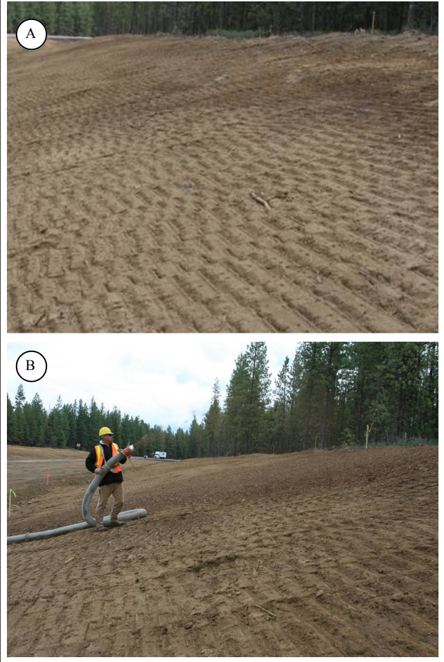
Figure 2. The trackwalking treatment (TW) shown in (A) stabilizes the soil through compaction and leaves the surface in a roughened condition. The trackwalking and mulch treatment (TWM) shown in (B) evaluated the effects of blowing a 2 cm (0.8 in) layer of ground wood mulch on a trackwalked soil surface.
