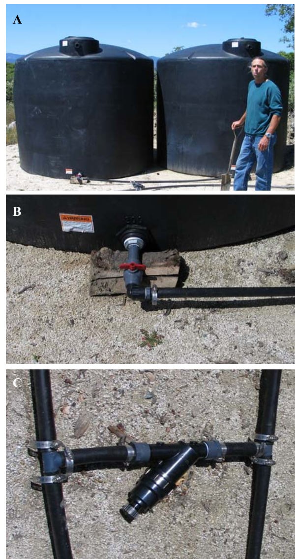
Figure 10.4.9. Large holding tanks are used for temporary drip irrigation systems. A simple on/off valve controls water to the gravity-feed system. Pressure release valves (C) are used to control water pressure on hilly sites.
